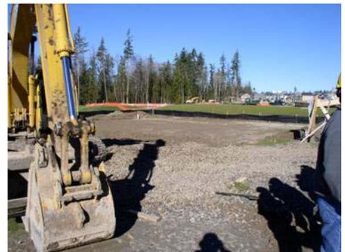
At Redmond Ridge, Quadrant Homes fences and protects areas of existing forest, as an amenity and stormwater filter. They chip land clearing debris. Then they grade to 12 inches below finish grade, stockpiling topsoil for reuse. Next step is to place rock pads for roads and driveways.
